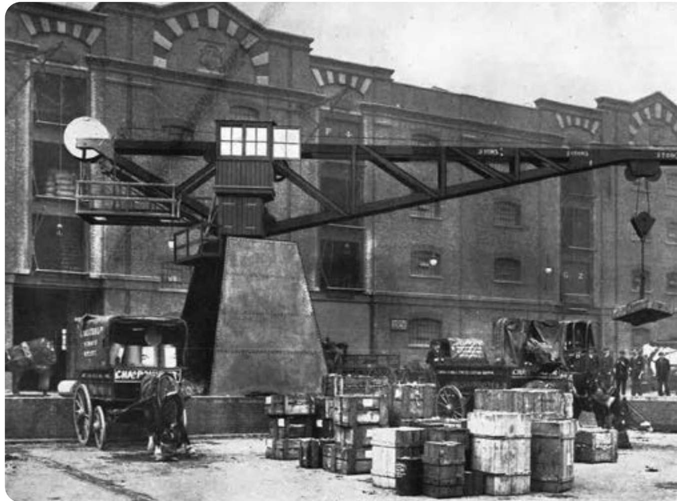
Joseph Stannah founded the business back in 1867, providing cranes and hoists to unload cargo in the docks of a developing London.
